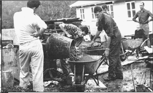
▲ Concrete pour for the first Water Tank under the first Kitchen and Dining Room.
