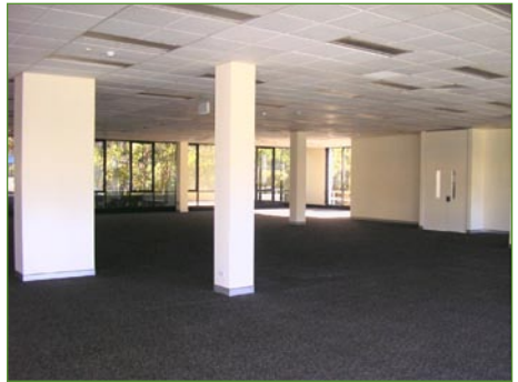
Inside view before fitout
