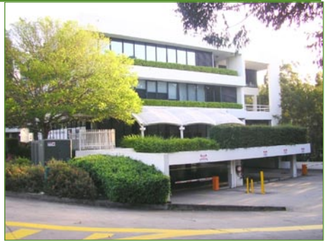
Northern end of building
